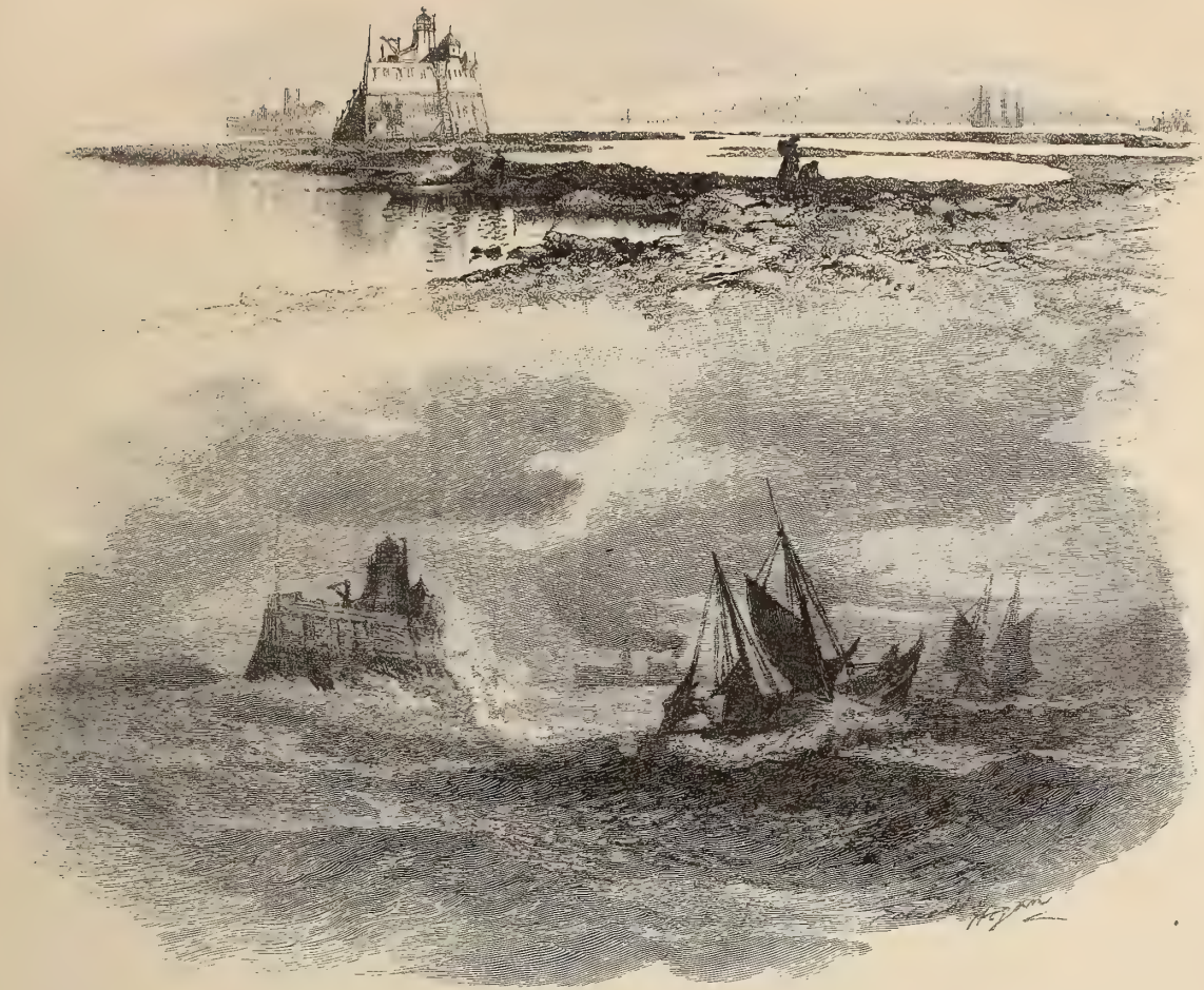
BEACON LIGHT, ST. JOHN, AT LOW AND HIGH TIDE.
